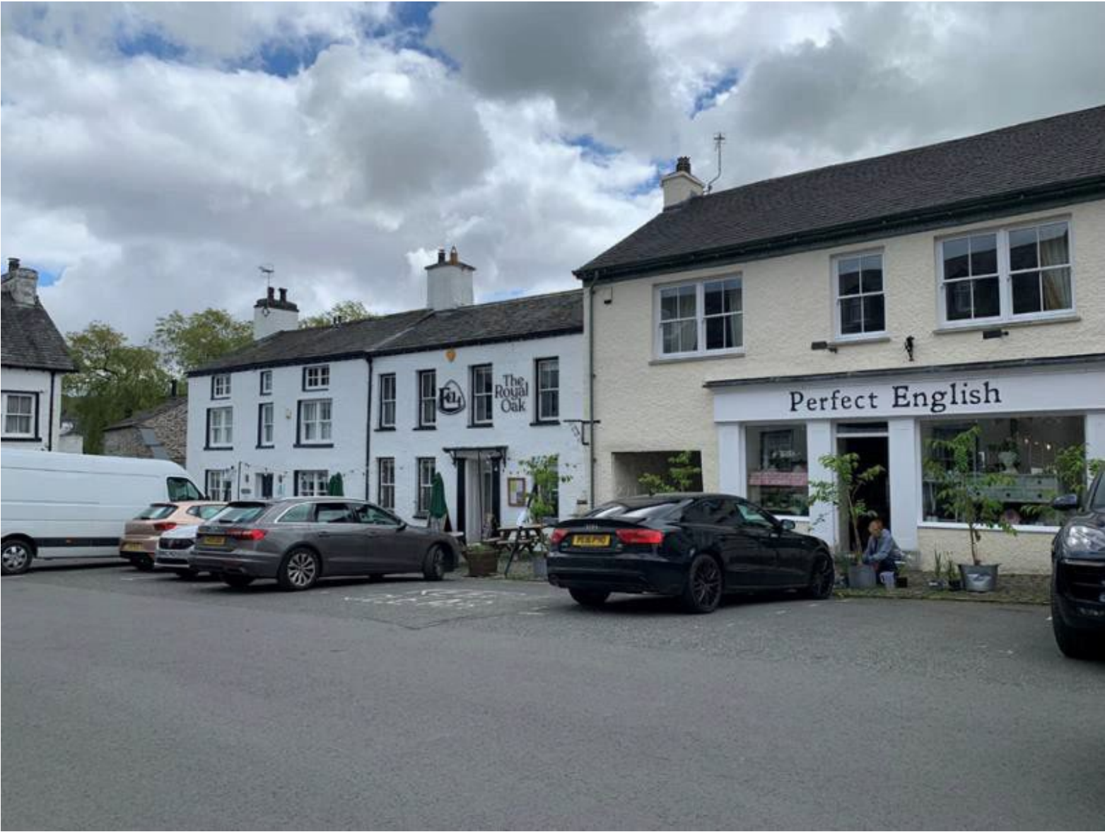
Figure 16: Rendered historic buildings in Cartmel in the Square. Use of render creates a sense of uniformity
